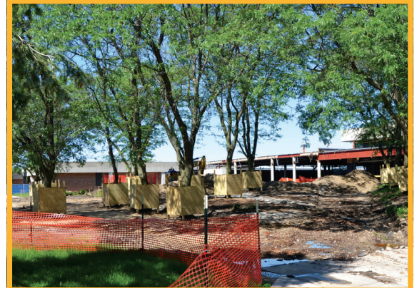
Ankeny's Rec Center construction project.
