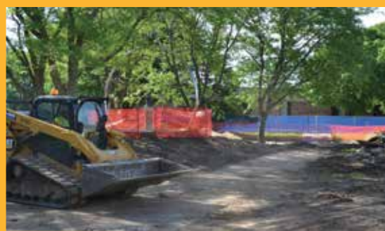
Starting construction on new Rec Center
